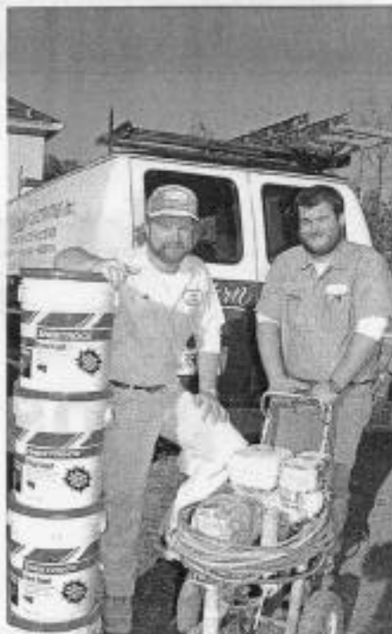
Mike Chandler (left) and Chris Chandler, of Modern Decorating, Inc., begin unloading materials for a drywall priming project at a commercial office building in Richmond, Virginia. Modern Decorating is a family-operated business, based in Richmond.
