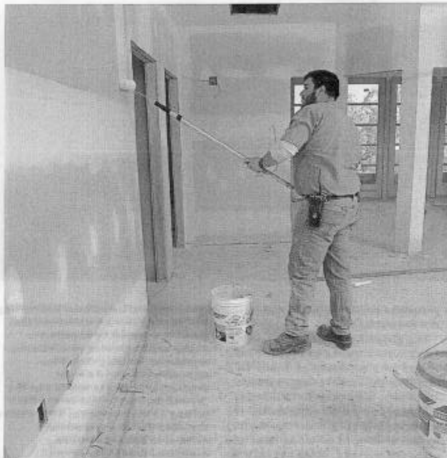
An equalizing primer will counter texture and porosity variations.
